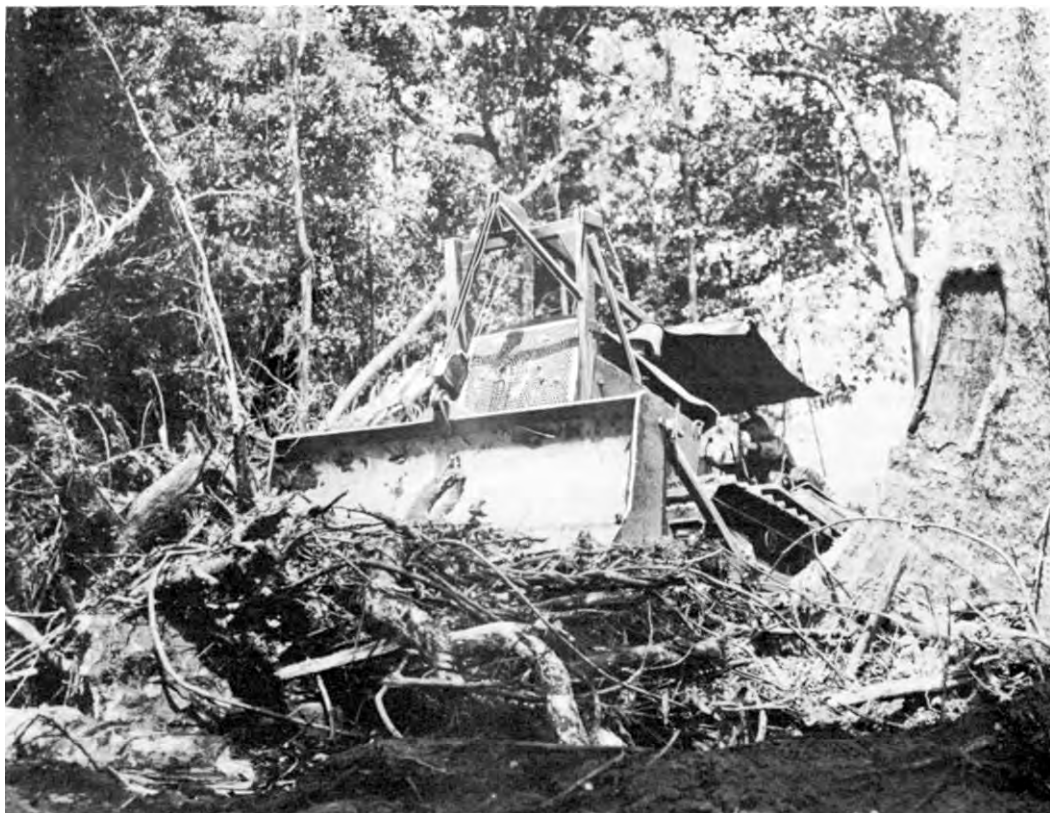
BULLDOZER CLEARING JUNGLE UNDERGROWTH for the construction of Mar Drome.
